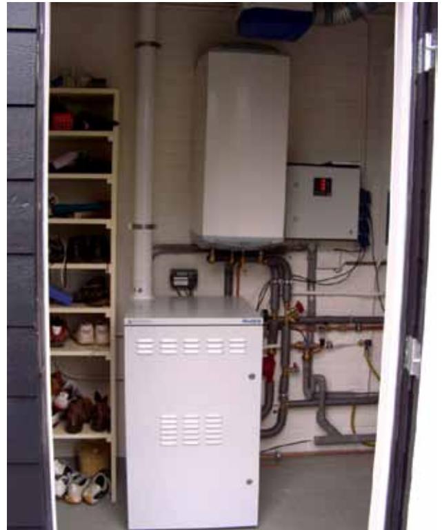
Şekil 3/Figure 3: Haren'de bir alan testinde CFCL Bluegen (Hollanda)/CFCL Bluegen in a field test in Haren (The Netherlands).
